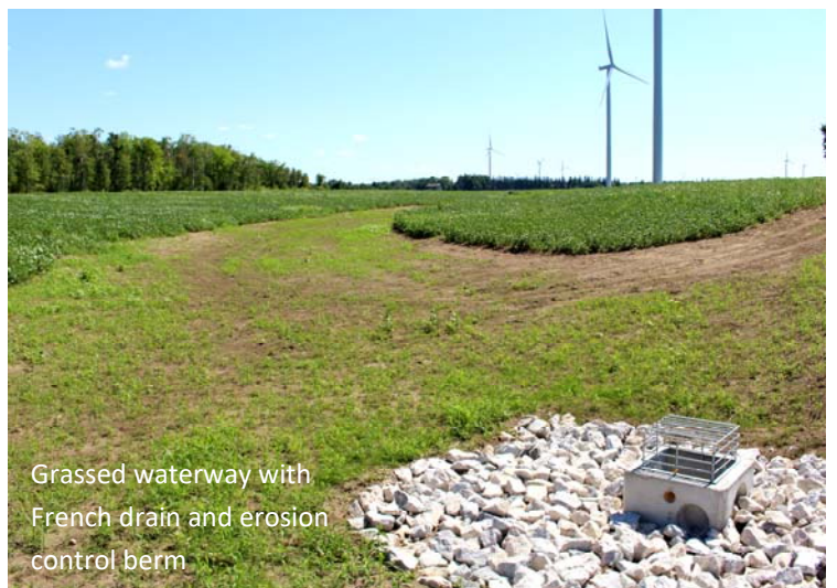
Broad-based berm with hickenbottom inlet
